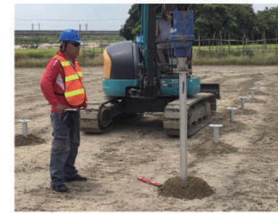
1 Ground screw installation
