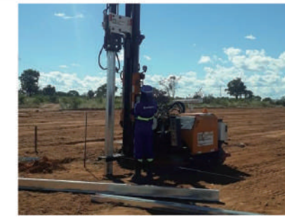
2 Ramming pile installation
