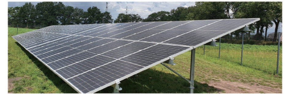
5 Fixing solar panel with mounting clamps
