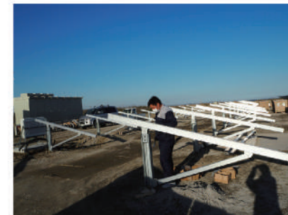
4 Fix Pre-assemble rack above ramming piles
