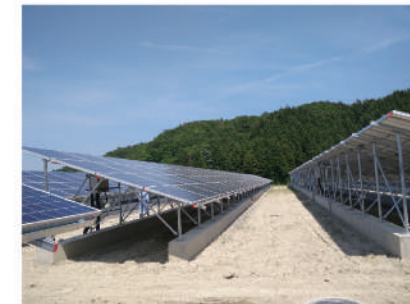
3.2 Fix rack above concrete base
