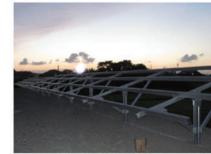
5 Install rails as drawing
