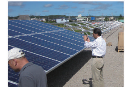
6 Fixing solar panel with mounting clamps
