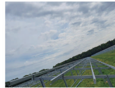
4 Install rails as drawing
