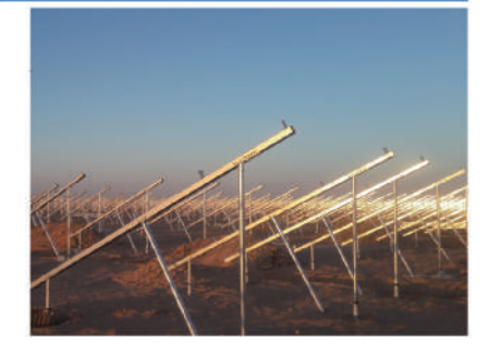
3.1 Fix rack above ground screw
