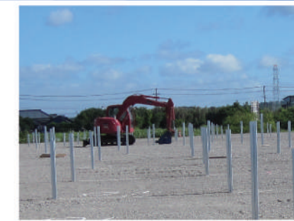
2 Ramming pile installation
