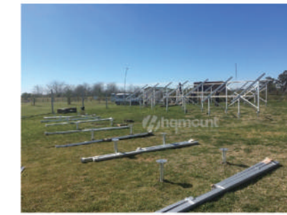
2 Unfold pre-assemble rack
