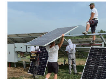
5 Fixing solar panel with mounting clamps
