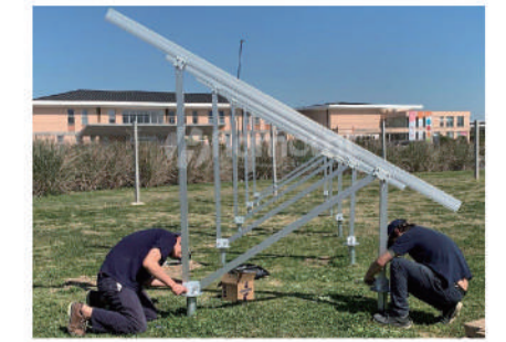
3 Fix pre-assemble rack above screws
