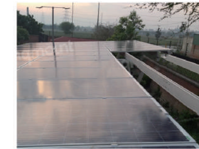
5 Fix panel with clamps
