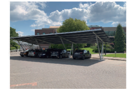
6 Installation is complete
