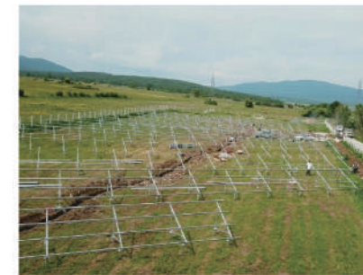
4 Install rails as drawing
