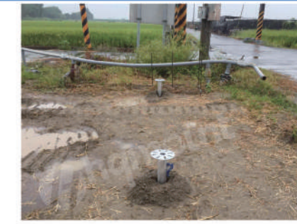
2 Ground screw installation
